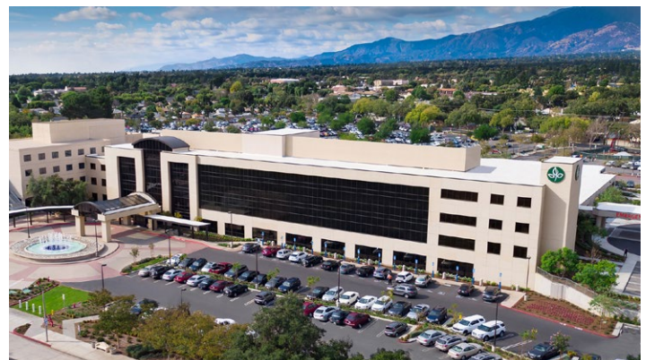
San Antonio Regional Hospital's new patient tower
