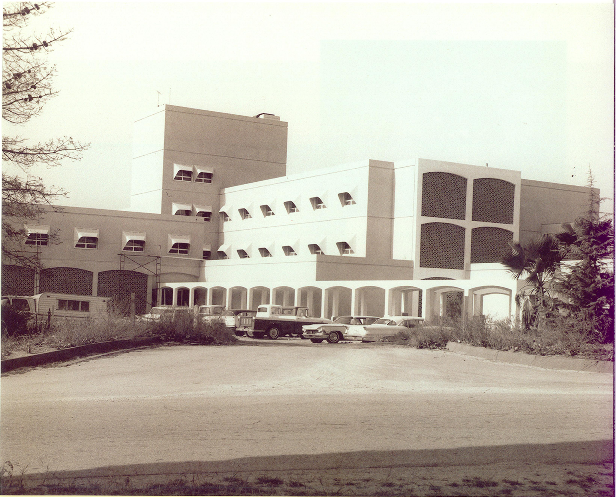
The Upland News featured the construction of the major hospital addition with the opening lines: "Early in 1964, San Antonio Community Hospital will open to the community a 95,000 square foot, four million dollar 'space age' hospital."
