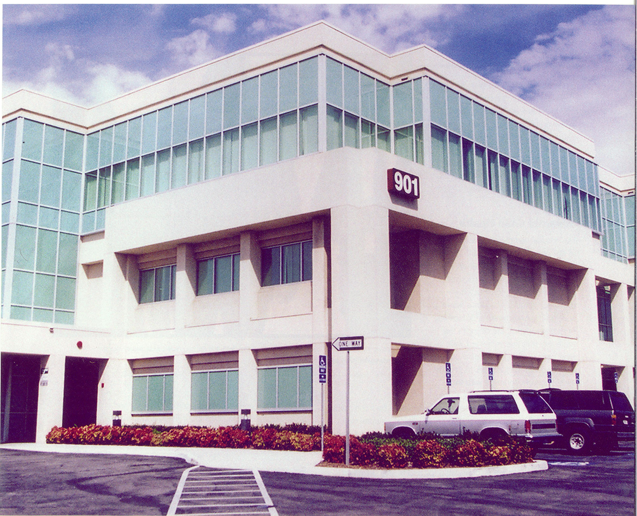
The medical office building at 901 San Bernardino Road opened in 1996.
